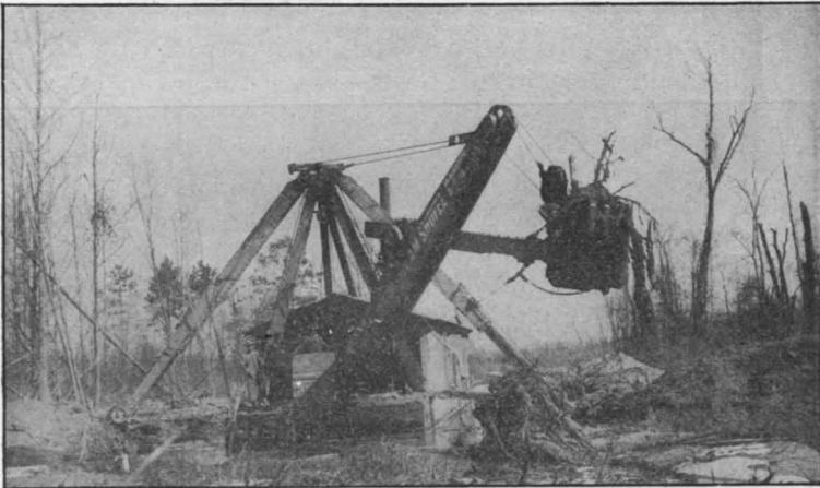
FIG. 2.—DREDGE DIGGING DRAINAGE DITCH THROUGH A SWAMP.
